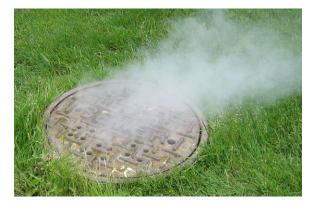
It is possible, although rare, that smoke could enter a residence through a drain trap which has dried out or some other plumbing defect such as an un-trapped washing machine drain.
